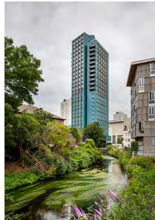
Breathing space. Mapleton Crescent - Metropolitan Workshop
