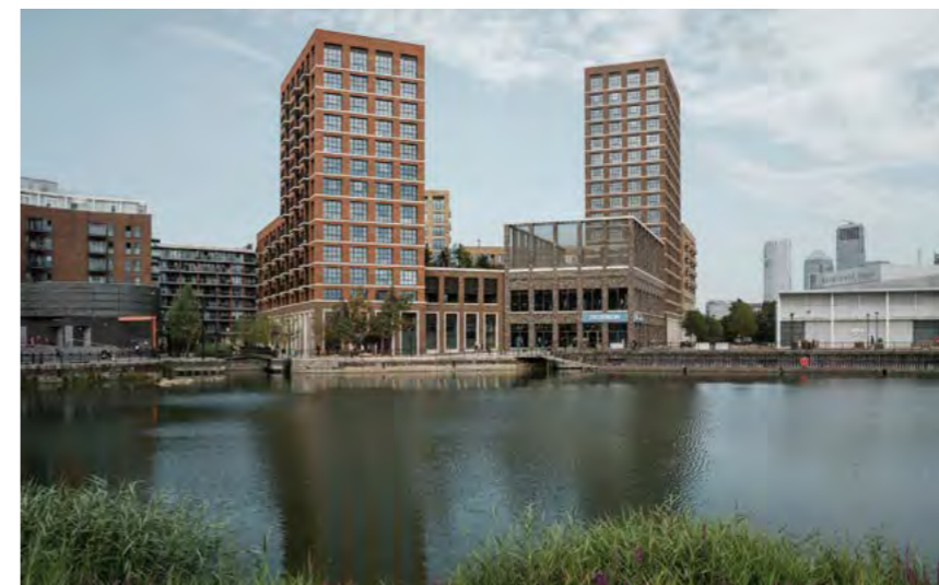
Porter's Edge - Maccreanor Lavington Architects.
