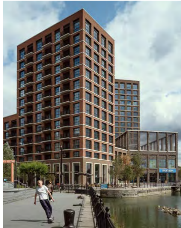
Porter's Edge - Maccreeor Lavington Architects.
