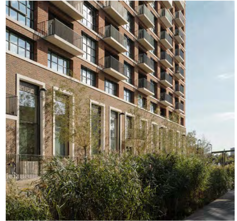
Porter's Edge - Maccreeor Lavington Architects.
